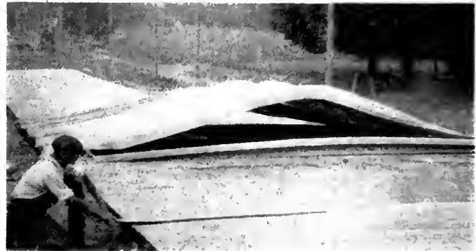
Movable canvas covered frame protects concrete.
